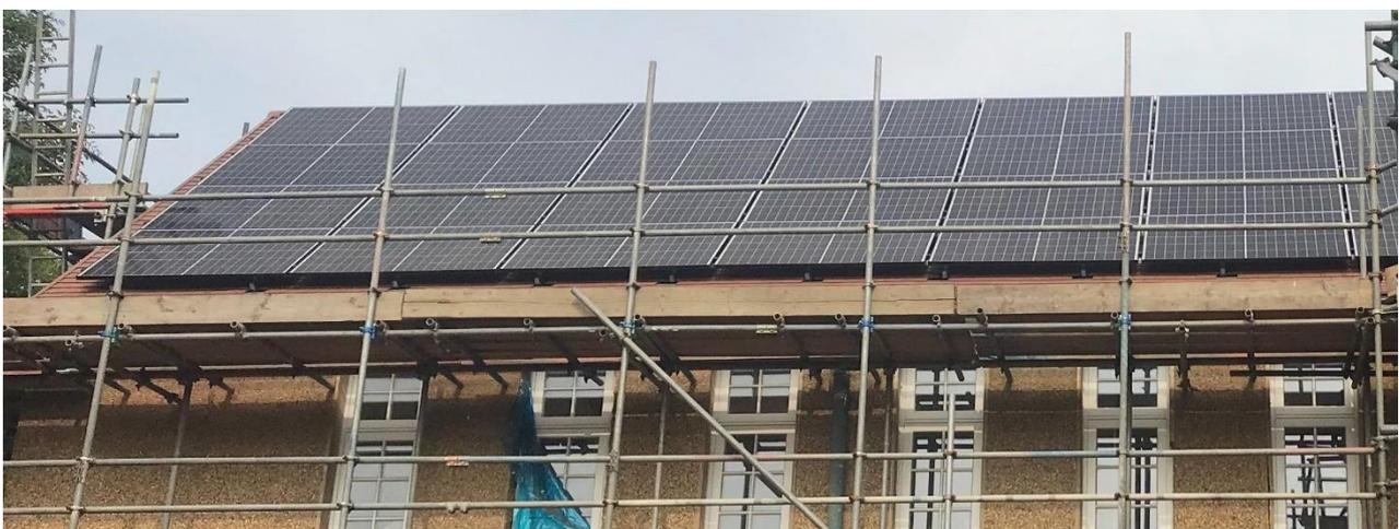
Photo voltaic solar panels on the roof of the main building take the solar energy from the sun and convert it into electricity which can be used inside the building.
